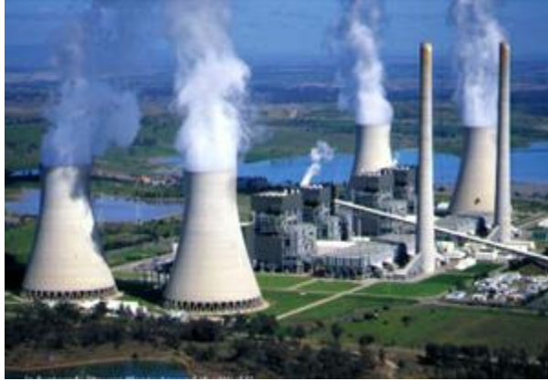
The Bayswater power plant in New South Wales is one of Australia's two largest coal-fired generating stations. (Photo courtesy Macquarie Generation)
